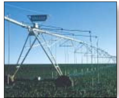
Irrigation Pivot —Irrigation monitoring reduces downtime and reduces costs.
