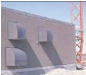
Remote Sites —Increase security and/or monitor power generators at detached or remote buildings.
